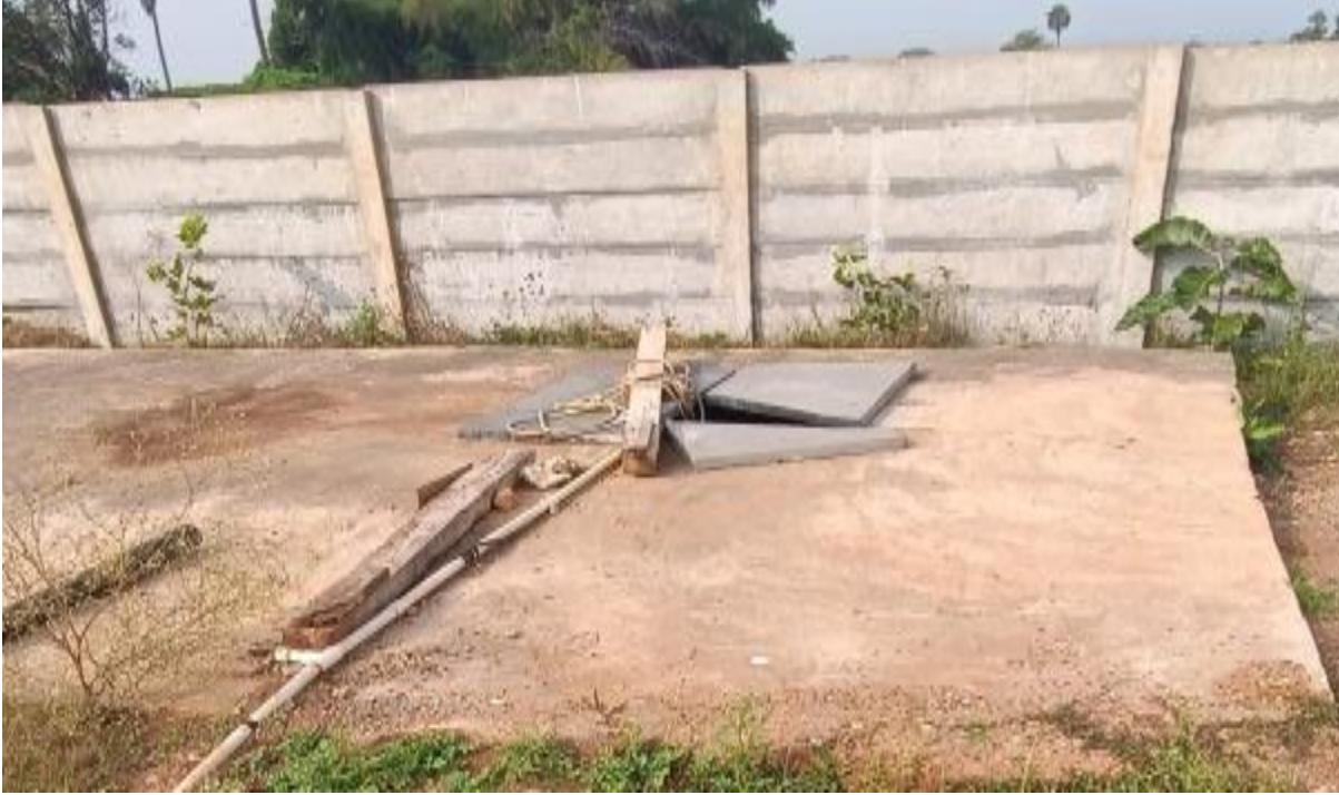
MISSION BHAGIRADA WATER STORAGE SUMP
